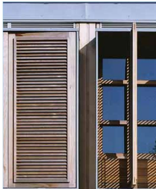
Use of external shutter shading to reduce solar gain to the inside of the building (© Peter Cook/VIEW)
