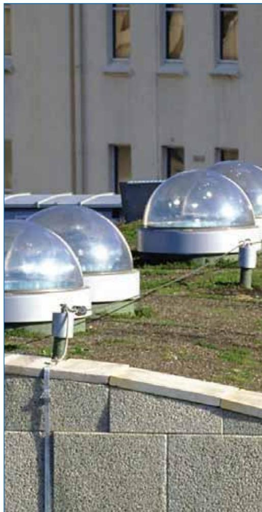
Green roofs at the Jubilee Campus designed to reduce storm run-off to drains
