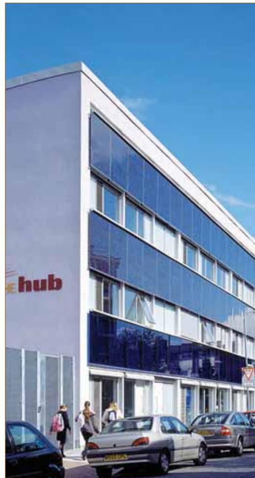
Photovoltaic Panels on the front façade of The Hub (© Dennis Gilbert/VIEW)
